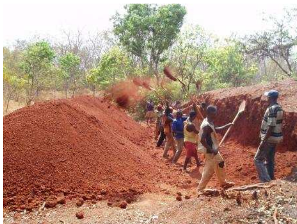
Local workers laying foundations for 48 km of road
