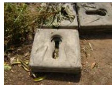
Concrete sanitary platforms
