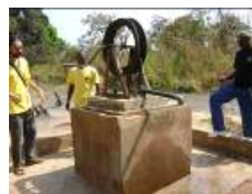
Rope-and-washer pump
